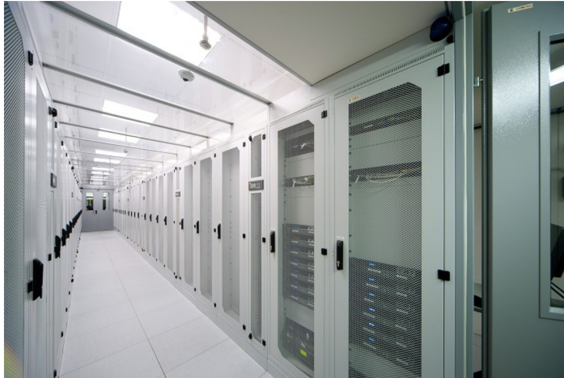
Server Room HC8 (2011)
